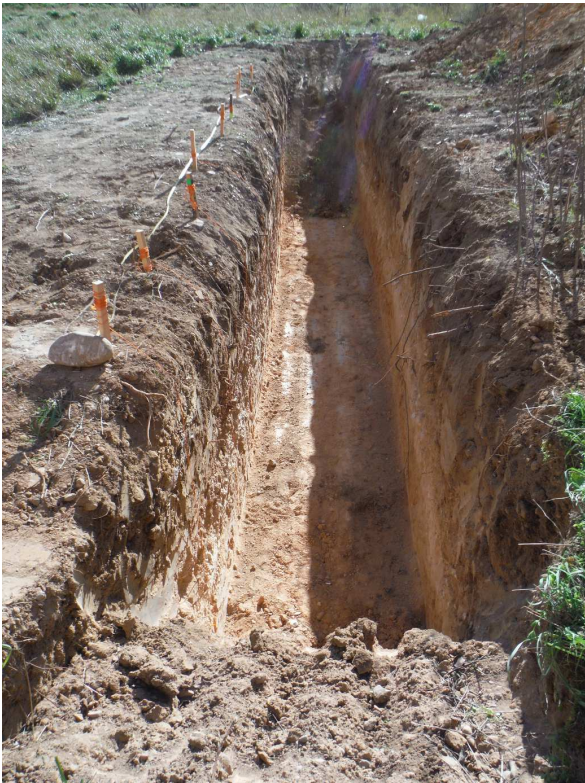
Vista general zanja
