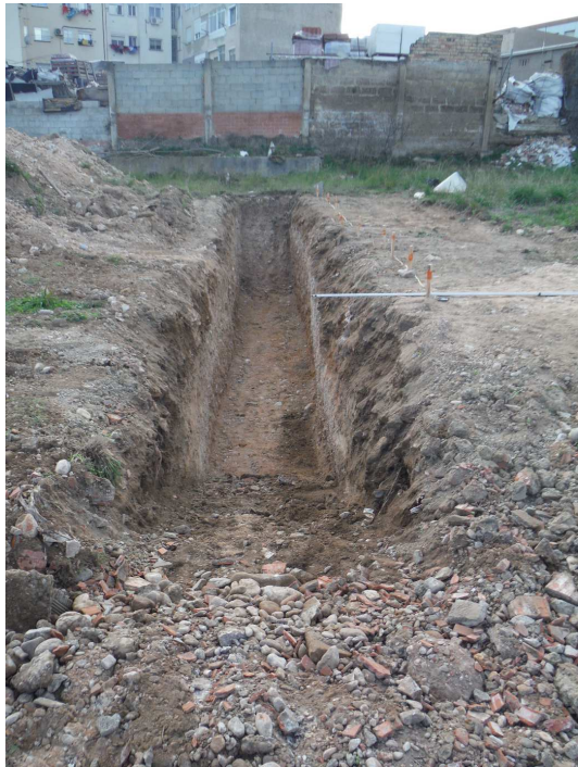
Vista general zanja
