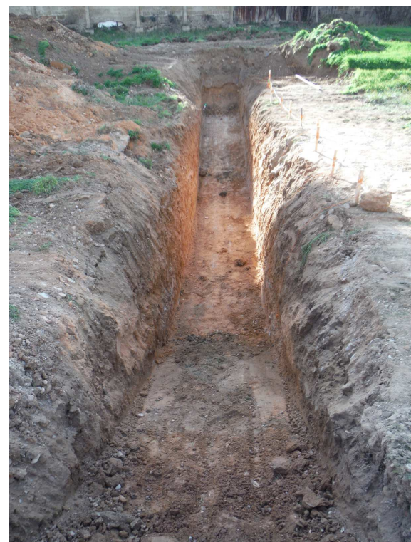
Vista general zanja
