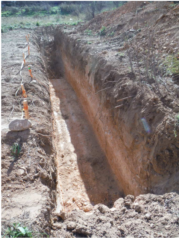
Vista general zanja
