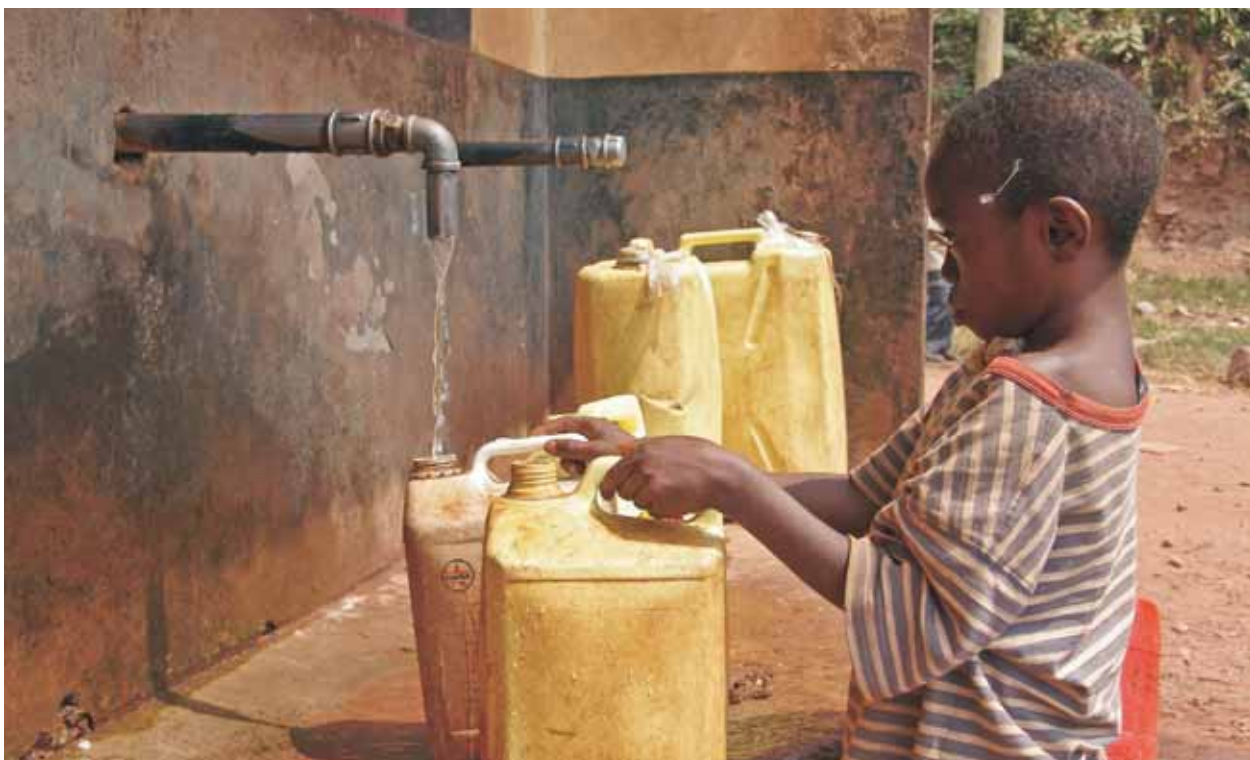
The main challenge facing Rwanda's water sector is a shortage of investment in human capacity building and infrastructure
