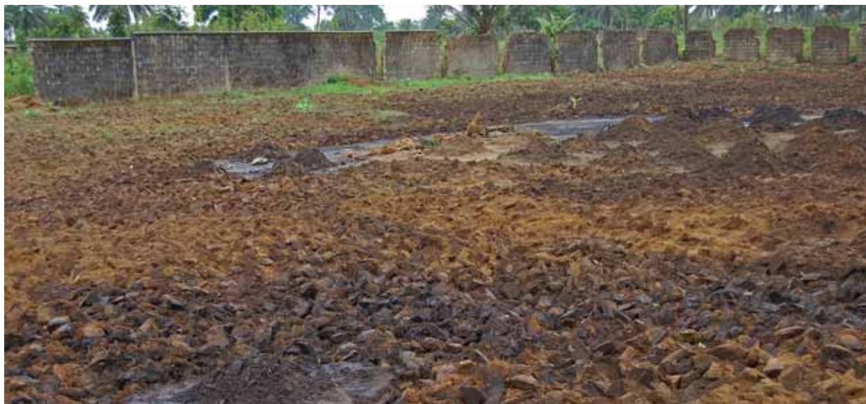
An Ogoniland site showing remediation by enhanced natural attenuation (RENA)
