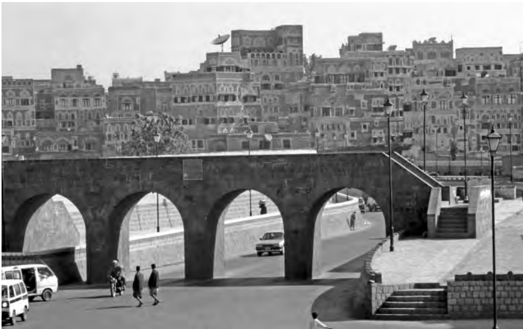
Photo 3.7: Roadway/flood channel Yemen. Source: Bill Lyons/World Bank
