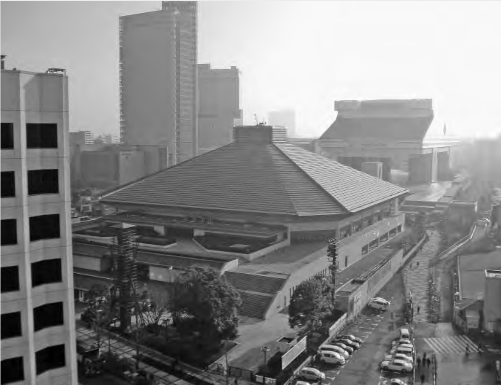
Photo 3.9: The Kokugikan sumo wrestling arena rain water harvesting system in Tokyo, Source: Japan Wikicommons
