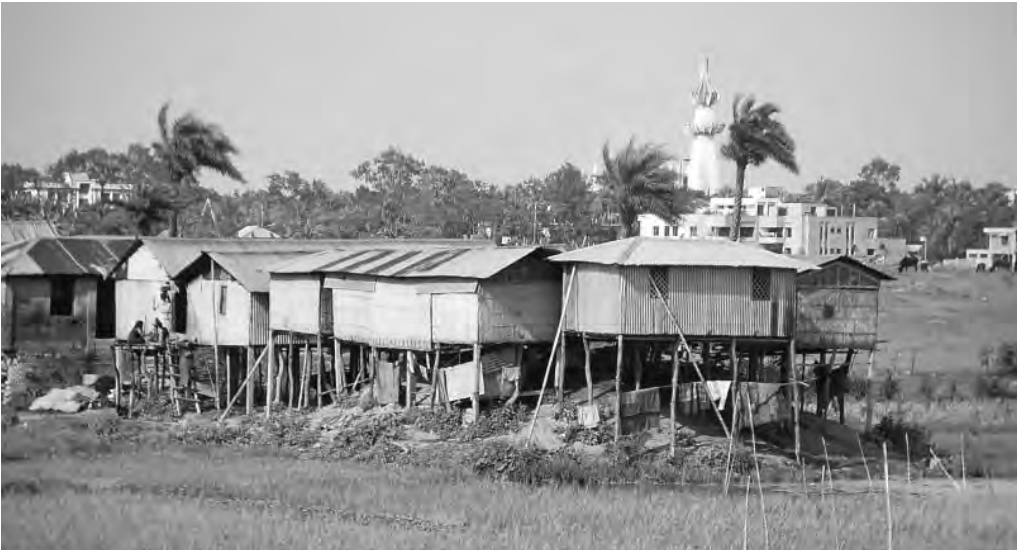
Photo 3.13: Houses raised on stilts to avoid flooding in Bangladesh. Source: Alan Bird.
