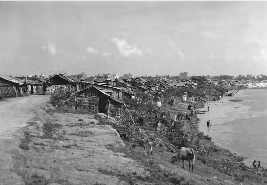
Photo 3.17: Multipurpose embankment with erosion. Source: Alan Bird
