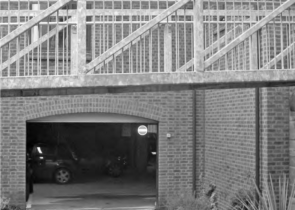
Photo 3.14: Municipal building in the UK with ground-floor garaging. Source: J Lamond.
