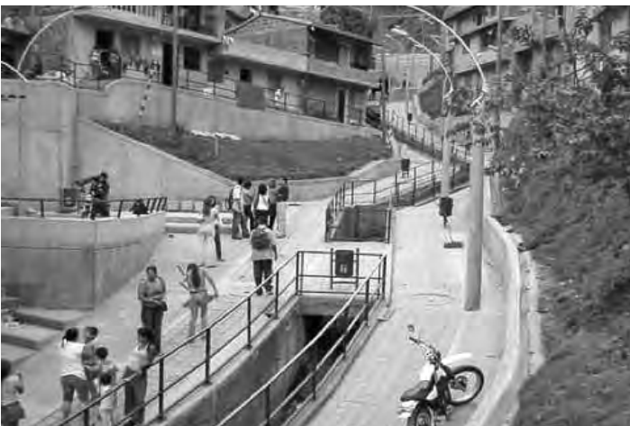
Photo 3.6: Reconstructed urban drainage in Acapulco, Source: UN-HABITAT
