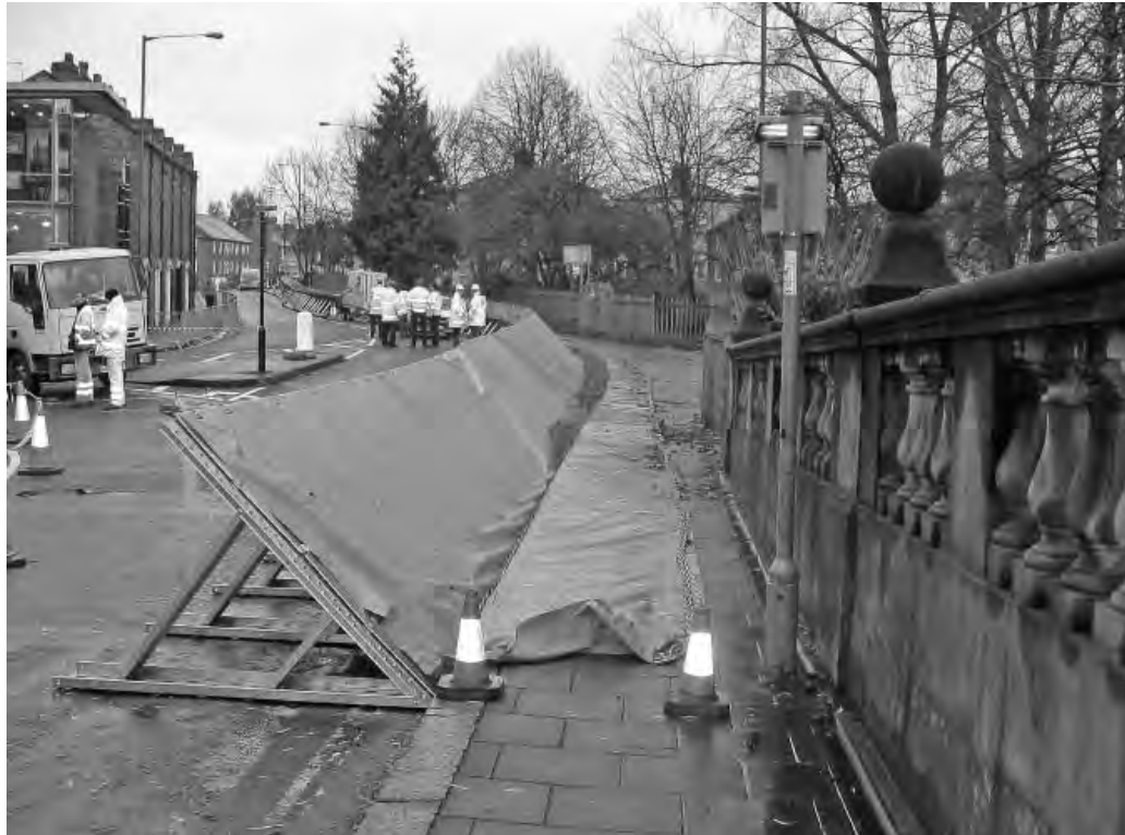
Photo 3.15: temporary flood barrier deployed. Source: J Lamond
