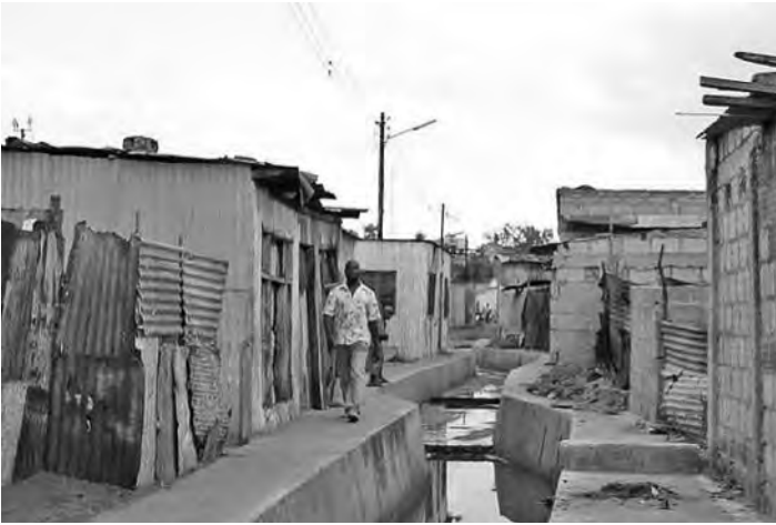
Photo 3.5: New urban drainage in Mafalala neighborhood, Maputo, Mozambique. Source: BBC News
