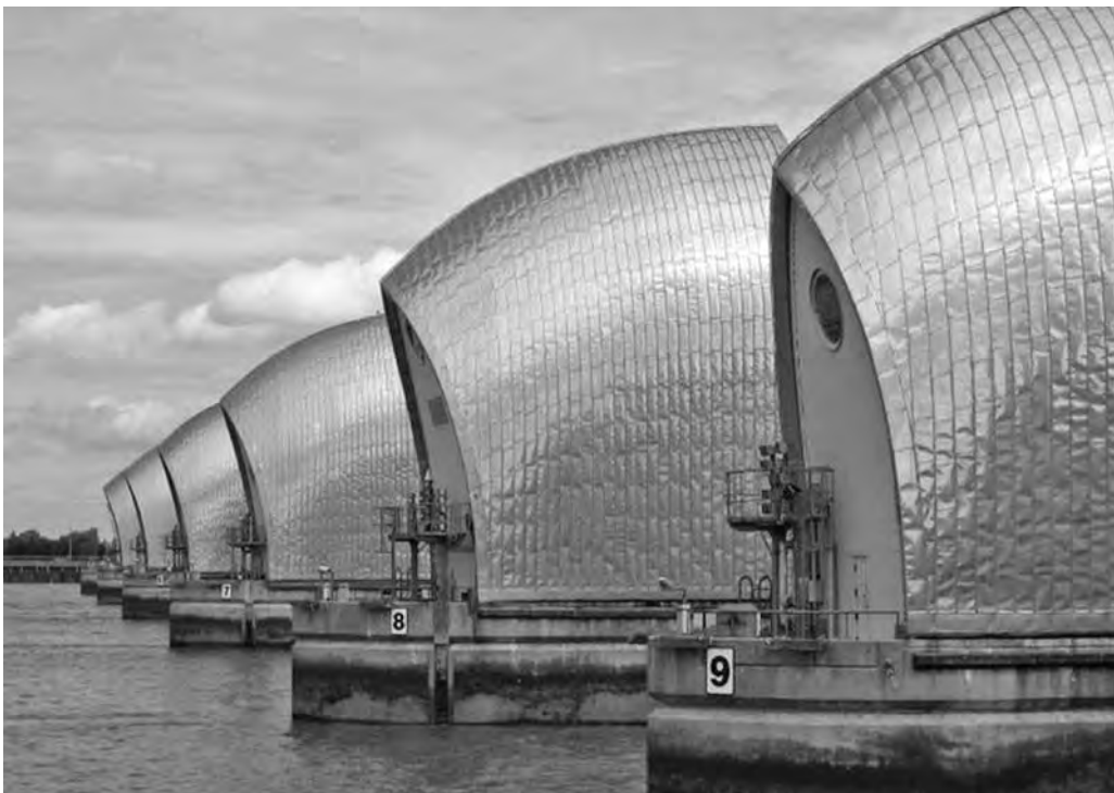
Photo 3.18: The Thames barrier, Source: Nick Dennison
