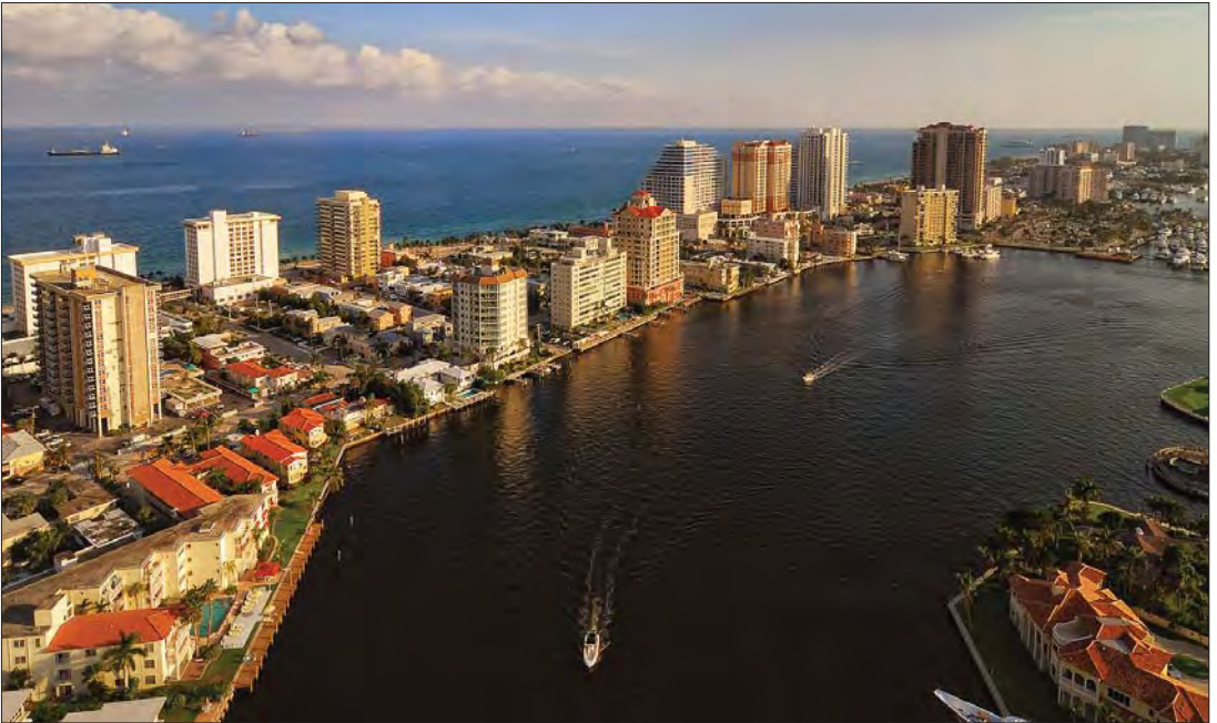
Cities will have to adapt coastal residential and commercial buildings to climate change impacts
