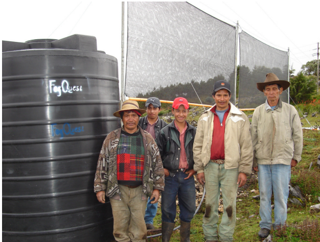
Figure 5: FogQuest Project, Tojquia, Guatemala, October 2006. Two large fog collectors and one 3000 liter tank provide water for one or two families.
